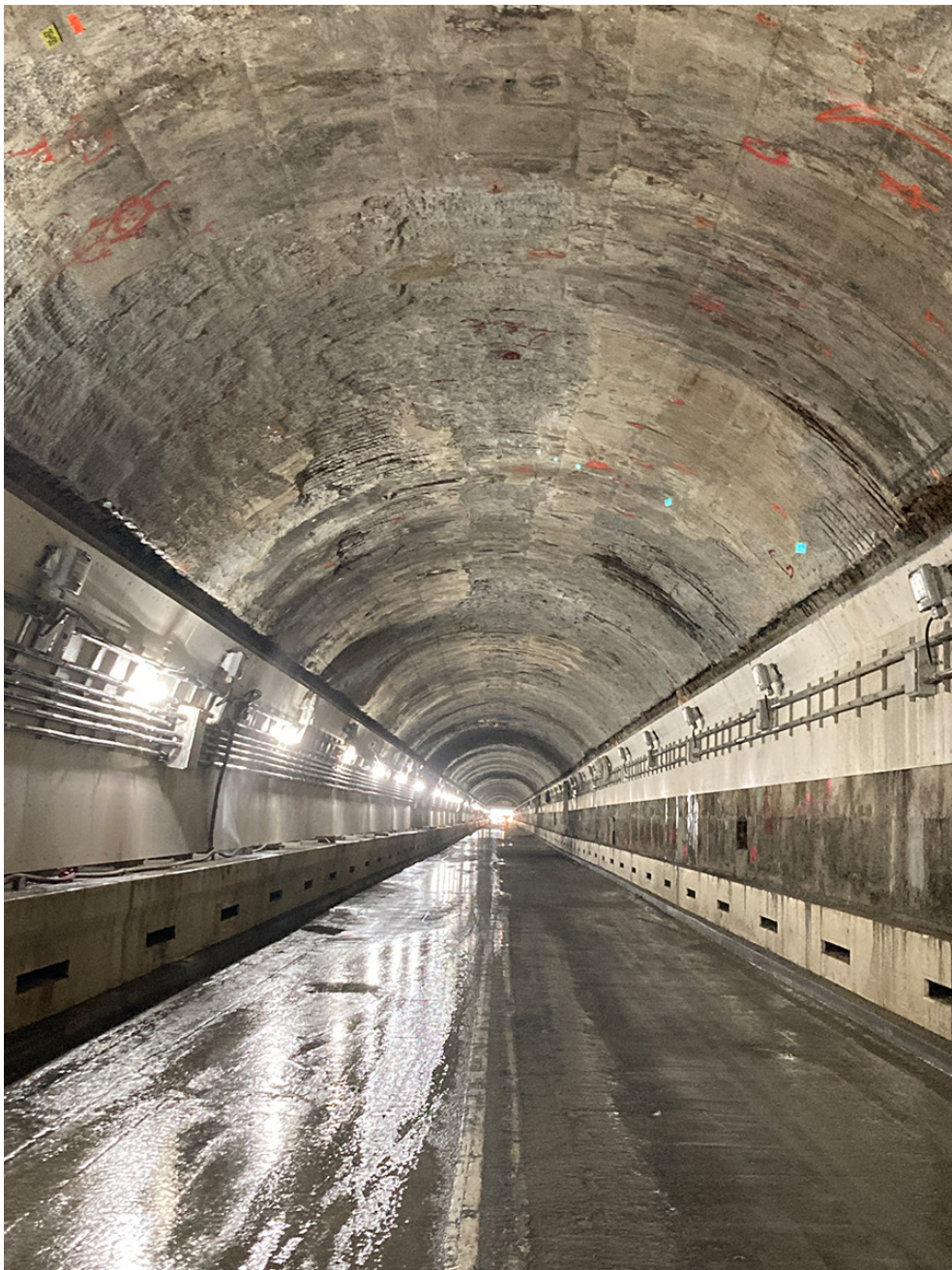
Existing tunnel ceiling, ready for precast installation
